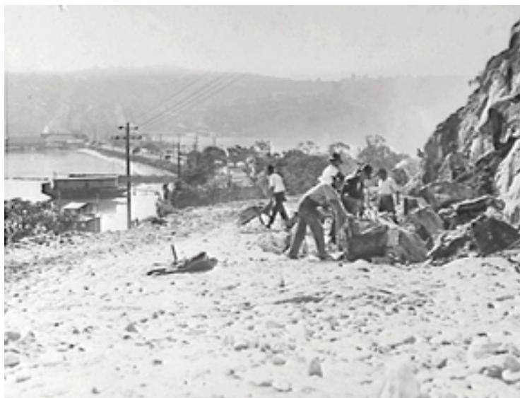
Excavating for the new Spit Road in 1922 (Mosman Library)
